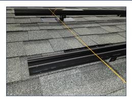
10 Tighten mount hardware as rail height and position are set at each roof attachment.
