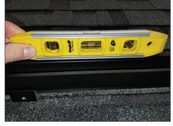
Run a string line or spare rail from the bottom rail to the top rail 6 and set desired pitch of the array by adjusting the top rail. Add Leveling Extension or spacer if needed (no more than 1 on 30% and 2 on 10% of attachments).
